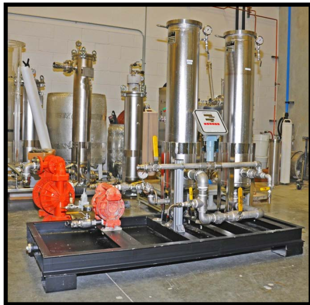
Air Driven Diaphragm Pump, Digital Flowmeter, 304 SS Vessels/Piping
